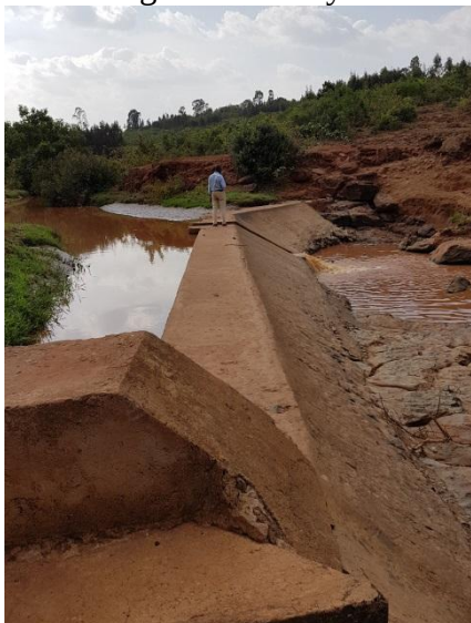
Cross wall for the capture of the river waters, Galda, Offa District (M. D'Agostini)
