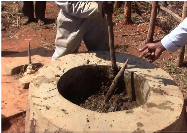
Stone basin for processing manure to produce biogas (M. D'Agostini)
