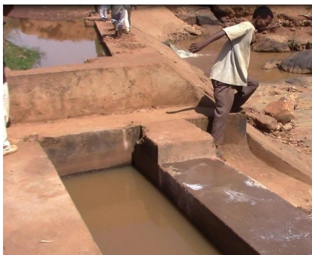
A weir from which the irrigation canal starts.
