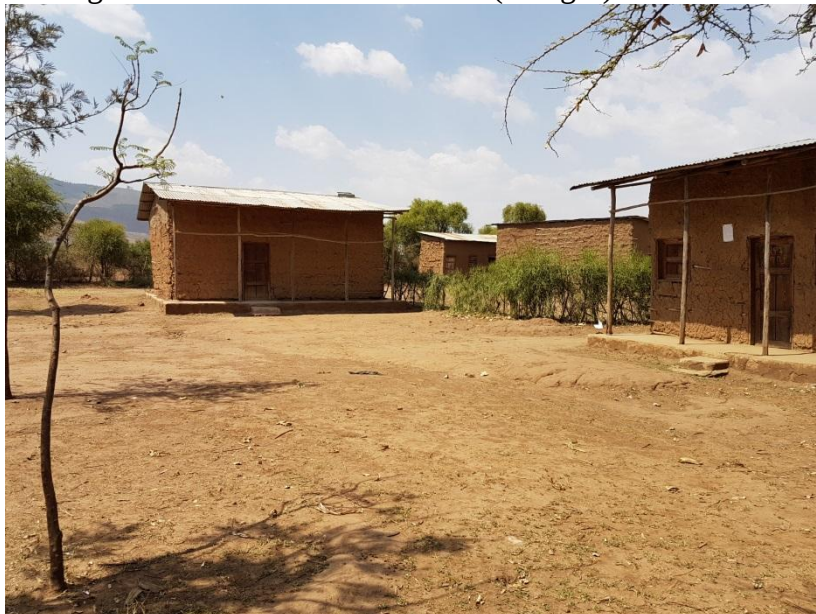
The headquarters of the "Town Hall" (on the right), the Local Manager's Office (Development Agent) of the District Office for Rural Development (left) and the school (in the background), in the Village of Fango Damot, in the Duguna Fango District
