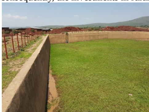
Dry basin for water collection, Bilate, Diguna Fango District (M. D'Agostini)
