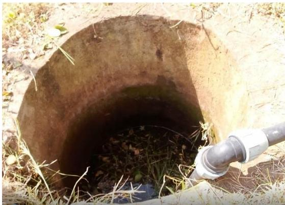
**The well built to collect water from a nearby canal, to be drawn by the Ampo Koisha pump powered by solar energy**
